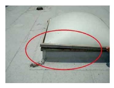
Also, over time the plastic domed panels can become brittle and very susceptible to cracks.
